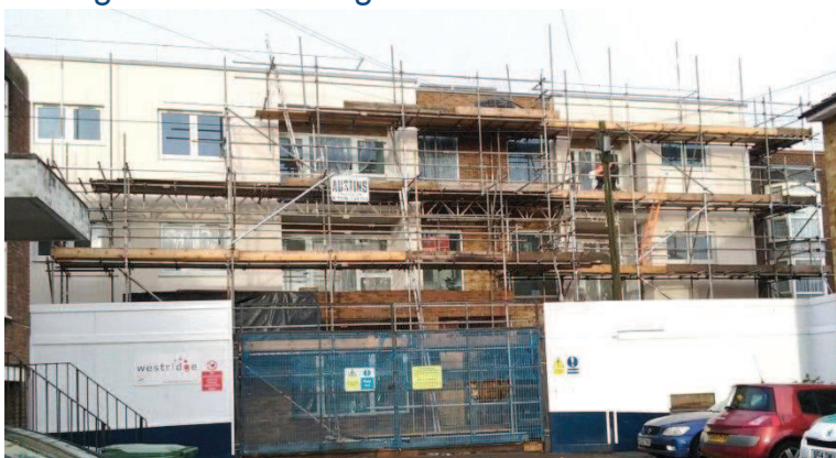
South side of the new Robert Lodge South block
